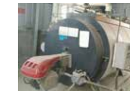
■ Air supply fan for boiler
